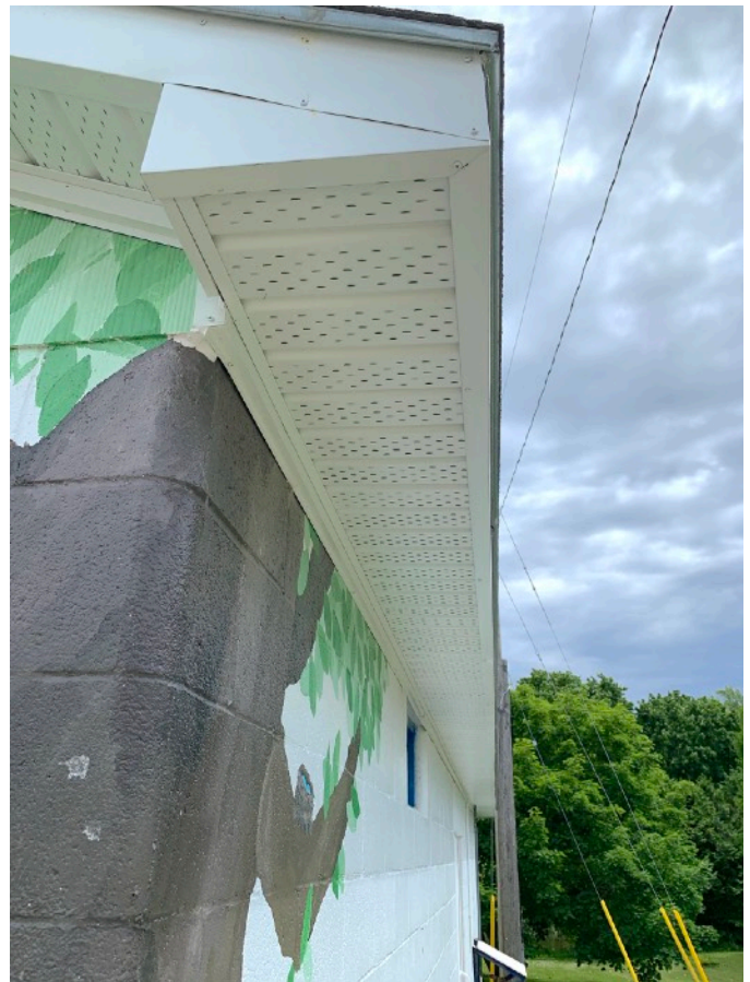
New vented soffits and fascia installed
