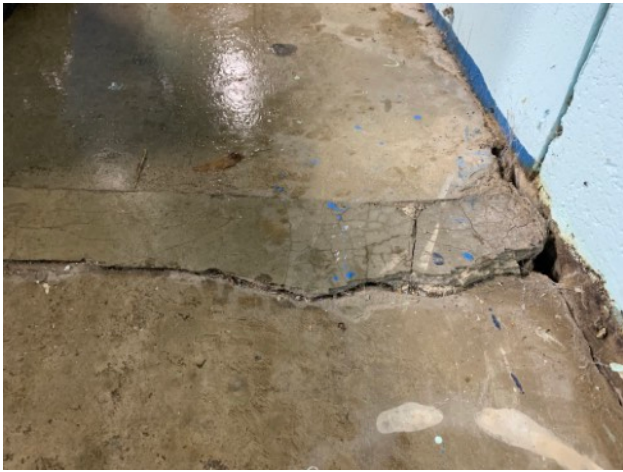
Large crack in main entrance
