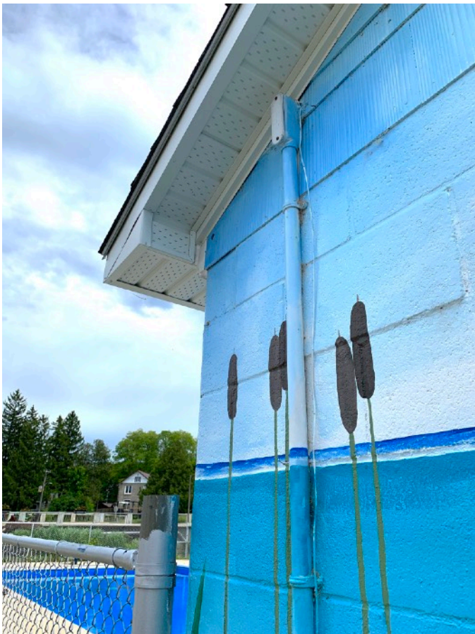
New vented soffits and fascia installed
