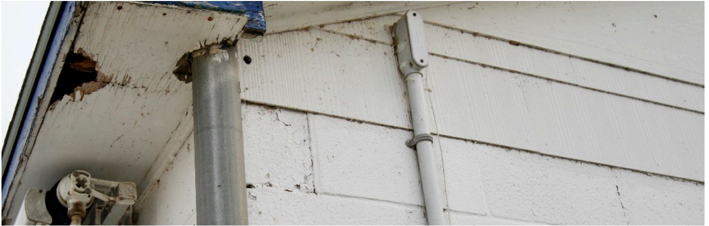
Existing Soffits - Rot and no vents.
