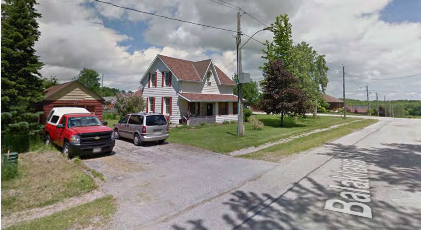
Image of Existing Structure
