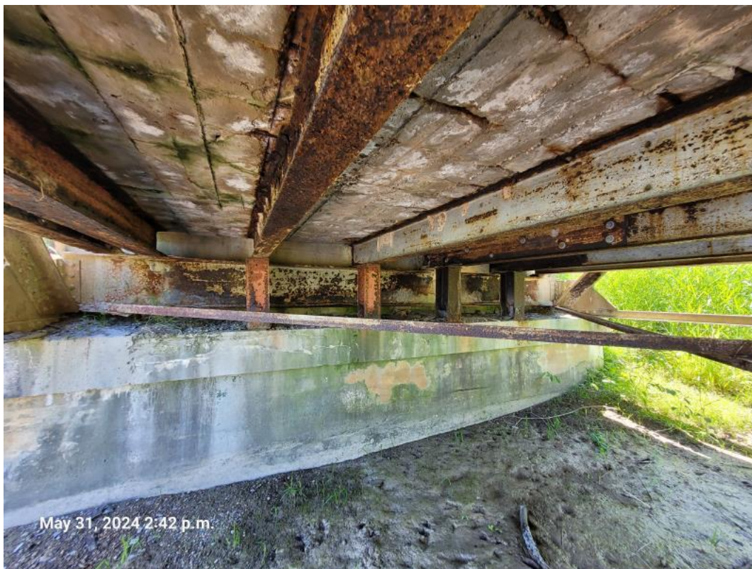
4-Soffit and South Abutment
