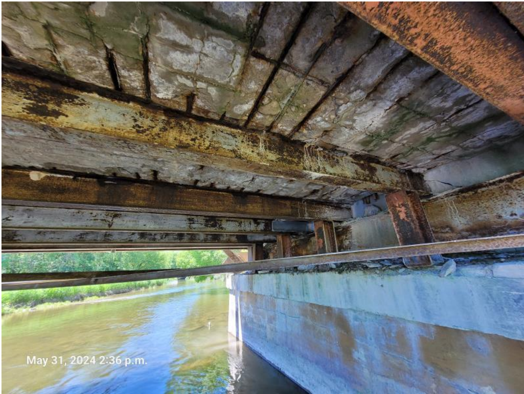
5-Soffit and Stringers at North End (1)
