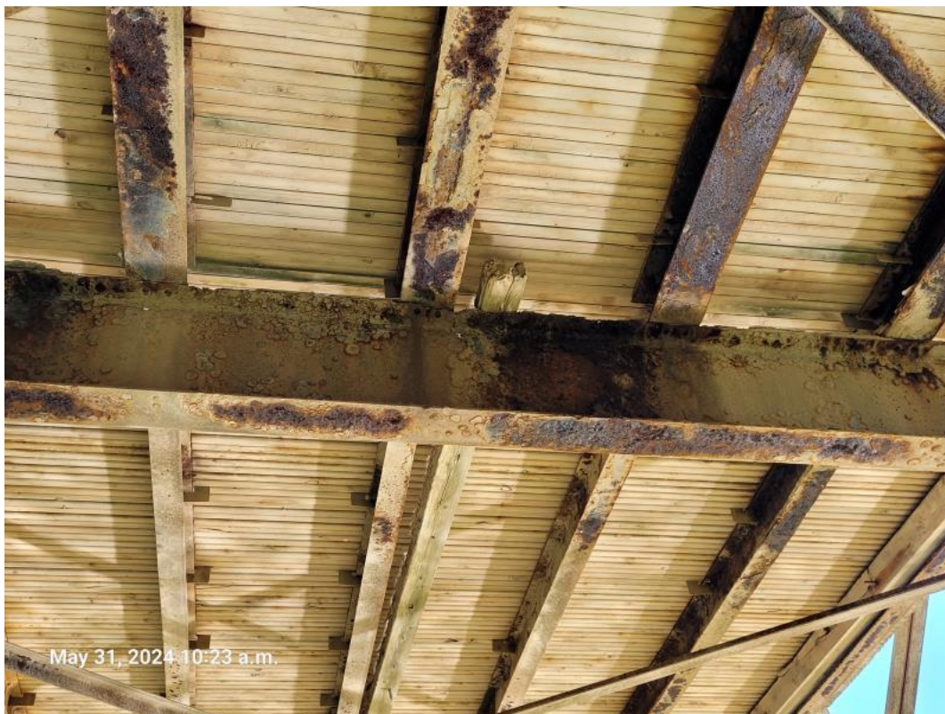
3-Soffit Looking North
