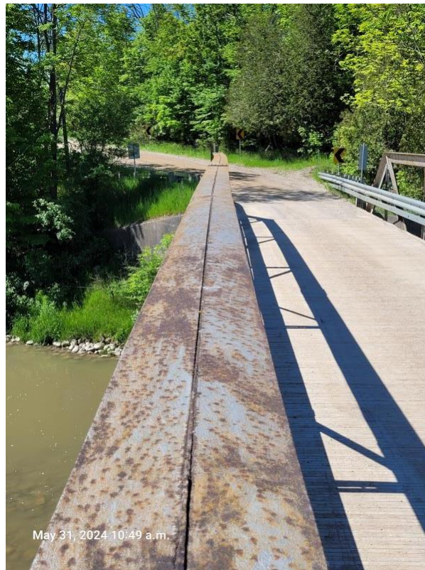
Top Chord-East Truss
