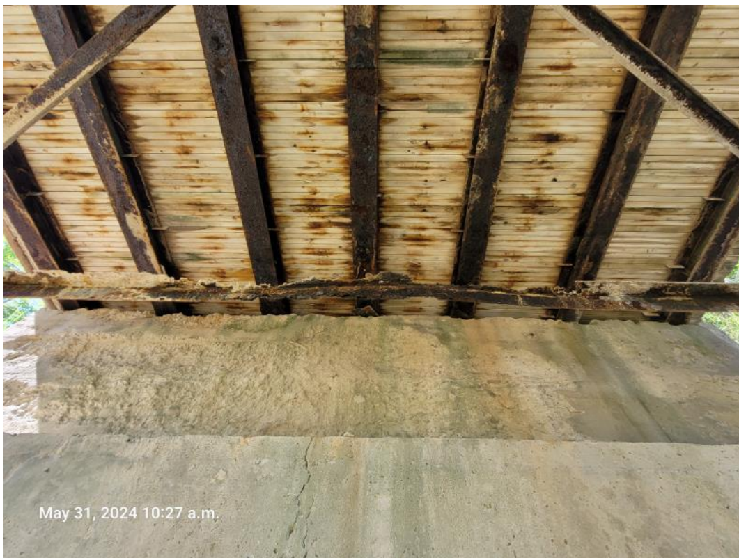
4-South Abutment and South Stringer
