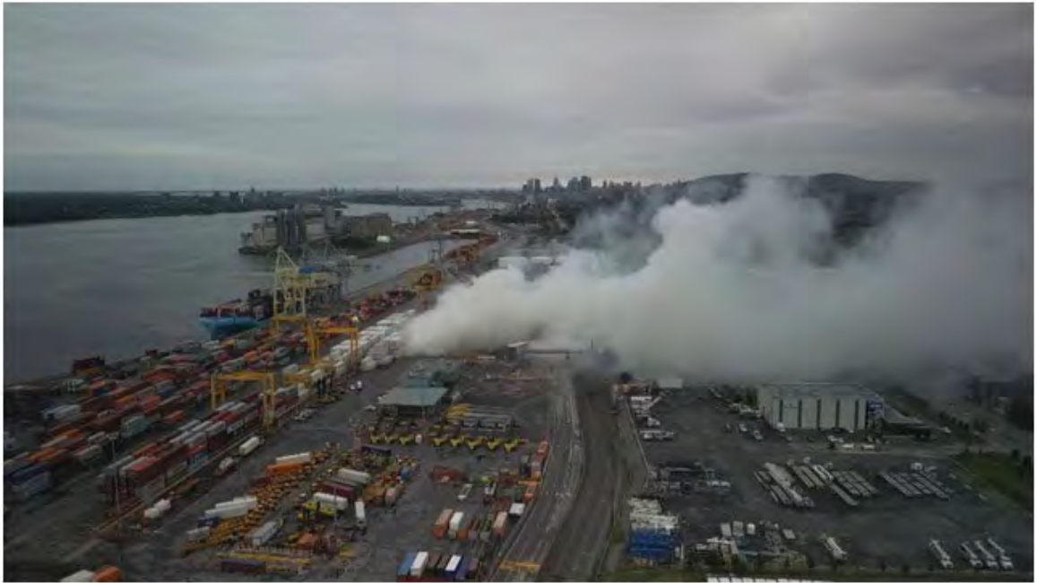
A fire at a shipping container at the Port of Montreal on Sept. 23, 2024. Global Montreal
